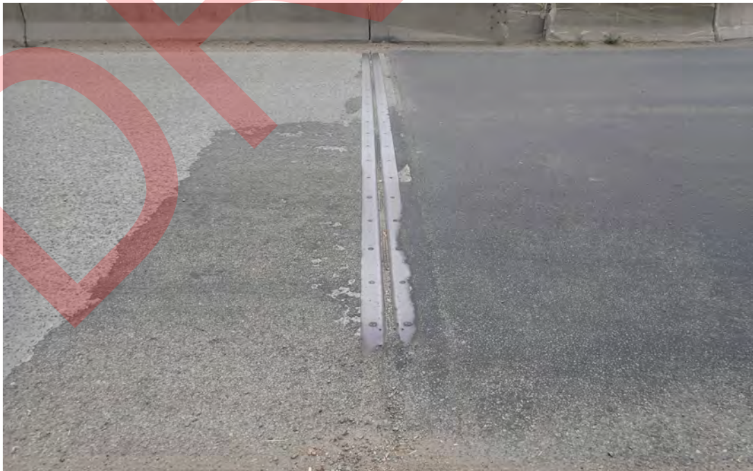
South abutment joint looking east.
