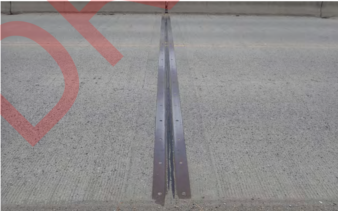
Joint at pier 8 looking east.
