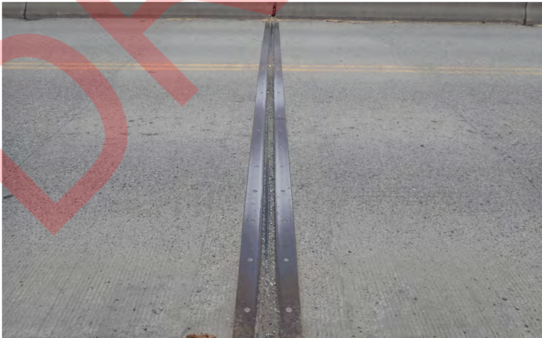
Joint at pier 20 looking east.
