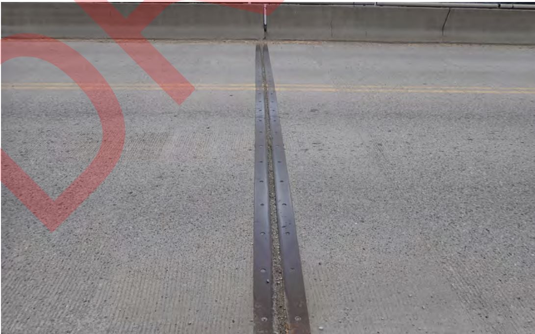
Joint at pier 16 looking east.
