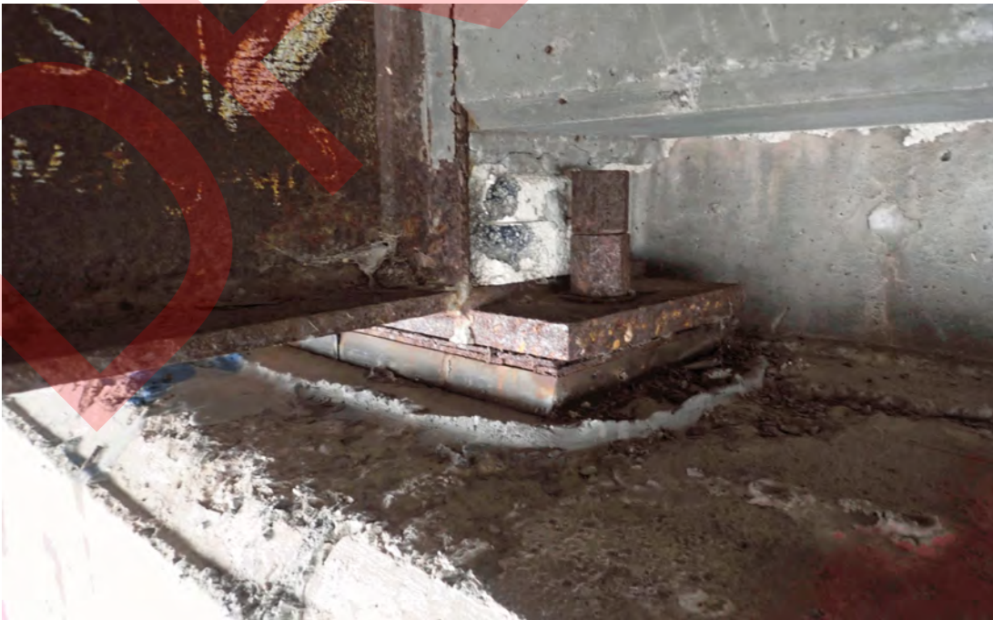
Typical condition of bearings at abutments.
