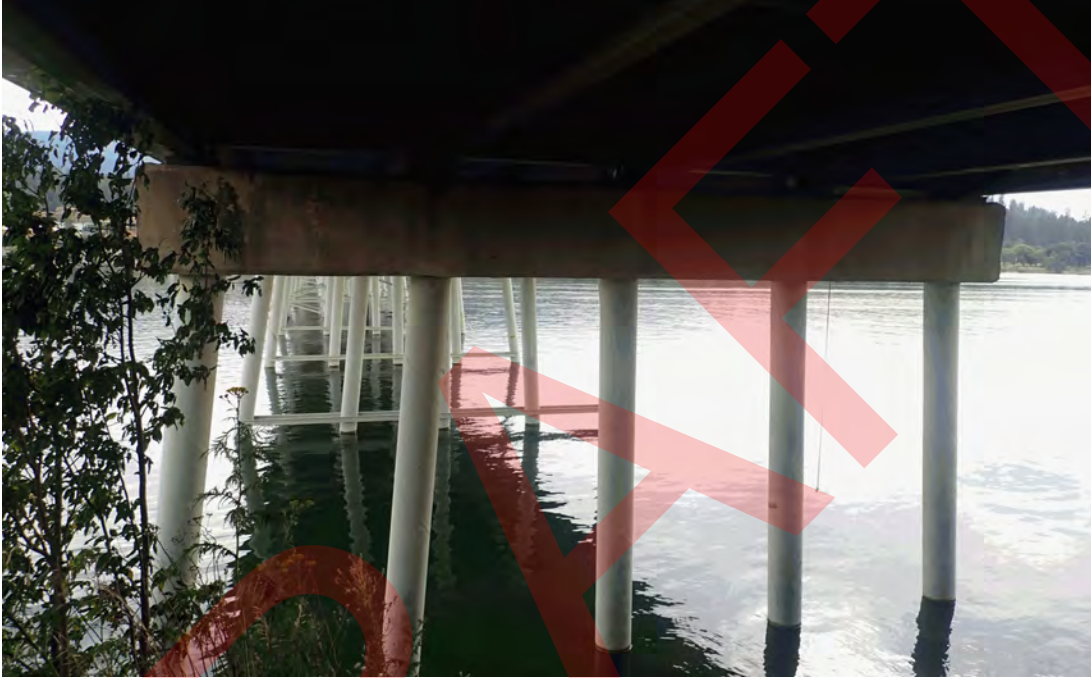
Typical pier and underside looking south.
