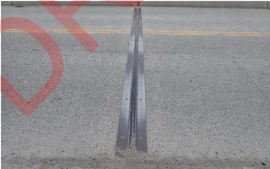
Joint at pier 30 looking east.
