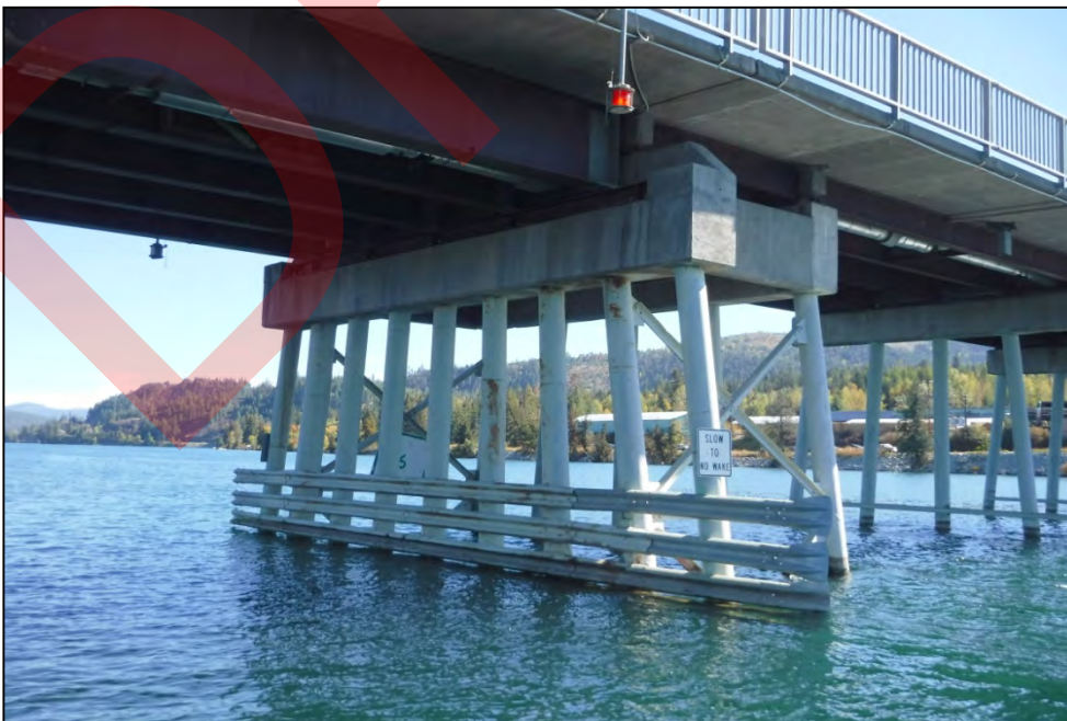
Photograph 4: View of Typical Tower at Main Channel, Looking Northeast.
